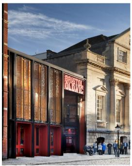
The south facing street facade has been conceived as a public art work, consisting of moveable sun shading shutters, operated by hand and incorporating the text both of the inaugural address given by Garrick in 1766 and a poem by former Bristol City Poet Miles Chambers. The text highlights the importance of the theatre's long history but looks forward to its role in the current and future life of the whole community.
